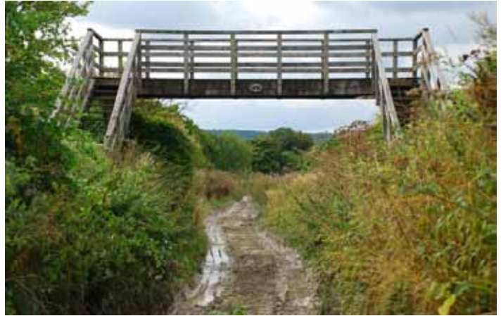
Bridge 4 in the summer of 2013 Mike Jackson © RGS-IBG Discovering Britain
