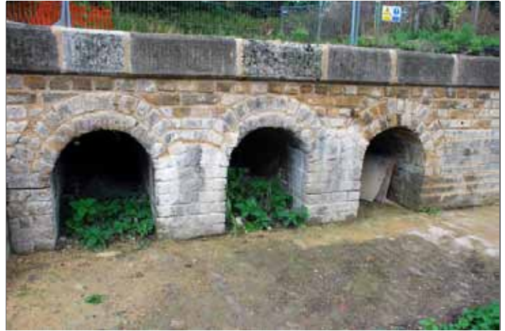
The base of Whitehouses pumping station Mike Jackson © RGS-IBG Discovering Britain
