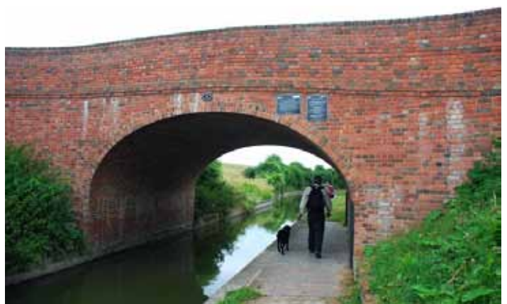
Top to bottom: the original Little Tring Bridge, the replacement under construction and the completed bridge © Wendover Arm Trust / Mike Jackson
