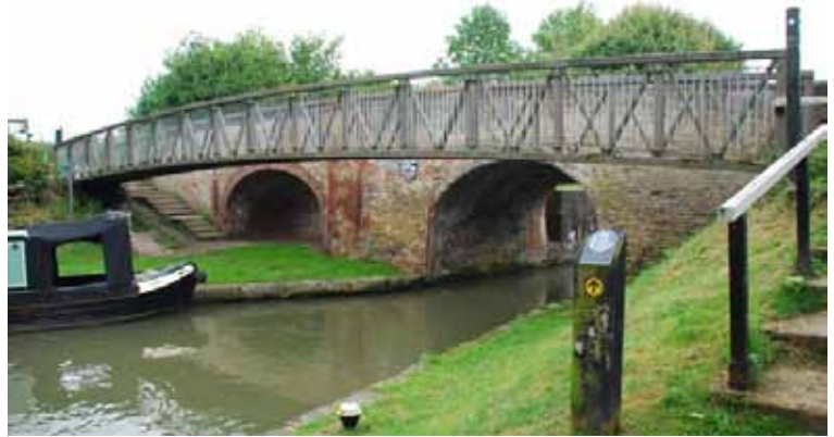
The double bridge with an arch over dry land Mike Jackson © RGS-IBG Discovering Britain
