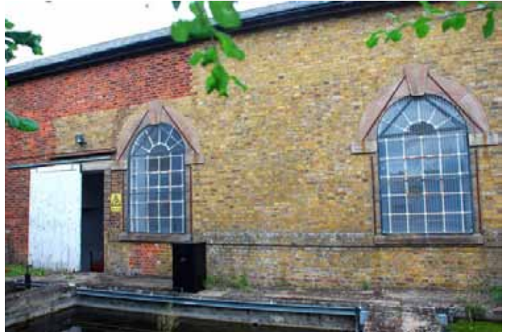
Tringford pumping station Mike Jackson © RGS-IBG Discovering Britain
